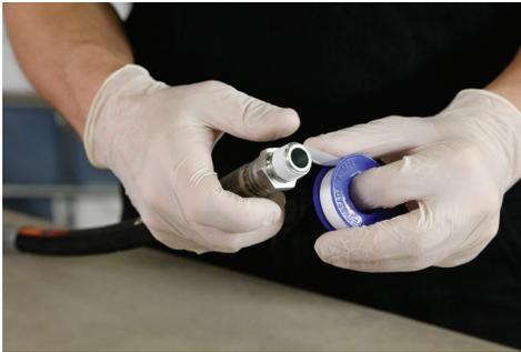
5) Dry the solvent from the ends of the mixing tube and whip hose and apply Teflon tape to the threads.
