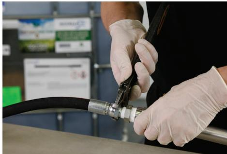
8) Attach the whip hose to the other end of the sample valve and tighten all connections.
